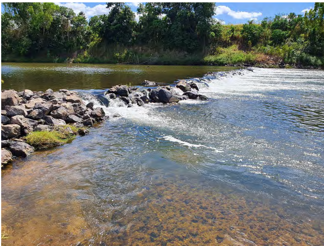
Figure 14 Rock weir on the Herbert River used as a pump site approximately 29 km upstream of the Herbert River mouth. Source: Fish Homes and Highways, Terrain NRM 2021.
